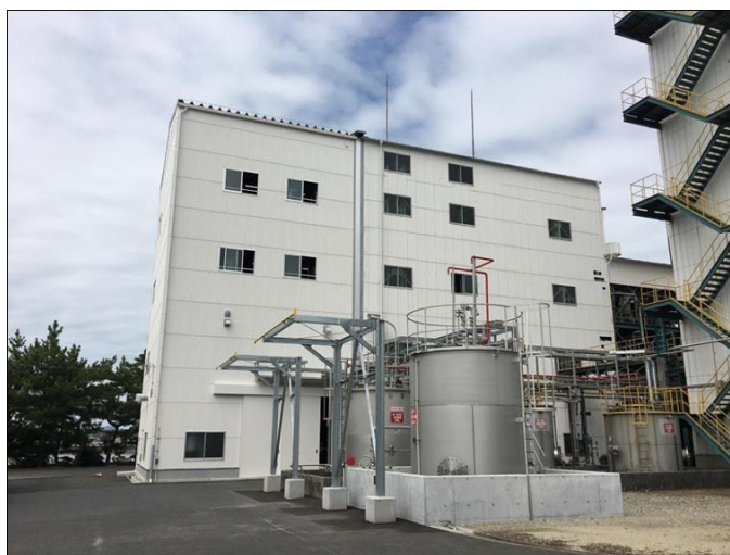
Manufacturing Facility for Gracia (NC-515)
