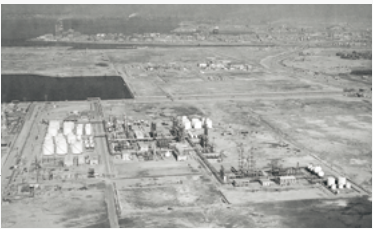
Nissan Petrochemicals Chiba Plant (1968)
