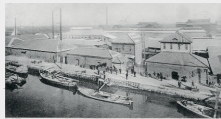
The land in Ojima 1-chome, Koto-ku, Tokyo, now known as Kamayabori, had been selected for its convenience in transporting raw materials and products. In 1888, the production of superphosphate (fertilizer) started.
