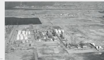
Nissan Petrochemicals Chiba Plant (1968)
