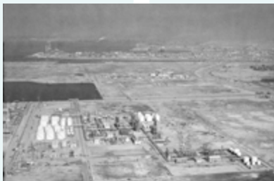
Nissan Petrochemicals Chiba Plant (1968)
