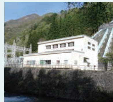
▲ Kuzuyama Power Station
