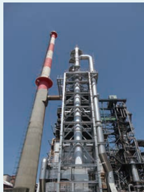
▲ Melamine heating furnace
