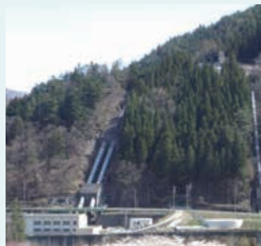
▲ Miza Power Station
