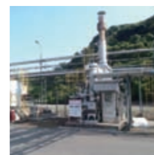
Exhaust gas combustion device
