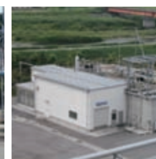
Discharged water treatment facility
