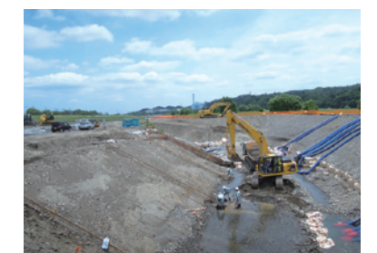
Tama river bank protection work against flood
