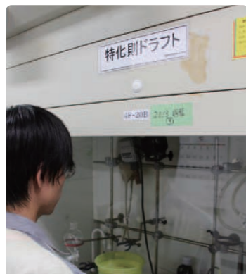
Exhaust ventilations for specific chemical substances
