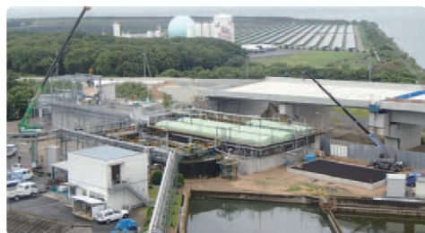
Construction work to reinforce waste water treatment facility
