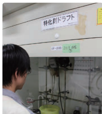
Exhaust ventilations for specific chemical substances
